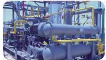
Raw material gas filtration, metering, pressure regulation Unit
